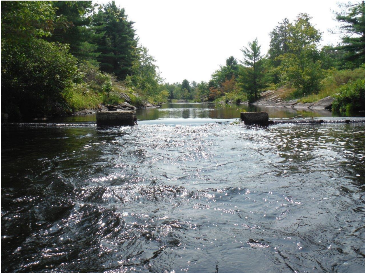
Head Lake Dam, located downstream of Head Lake along the Head River (August 2016)
