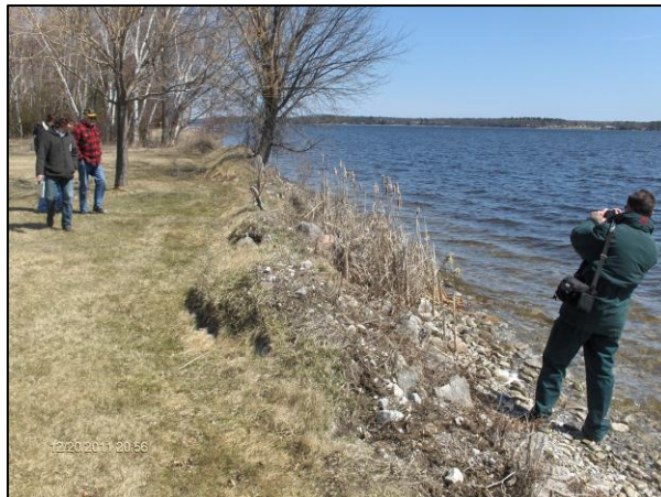
Effects of ice heaving on a developed shoreline (Victoria Place, 2011)
